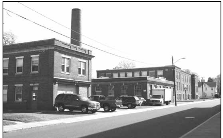
The three Bennet buildings at the center of the controversy: a firehouse, boiler plant, and Cheney Building.
