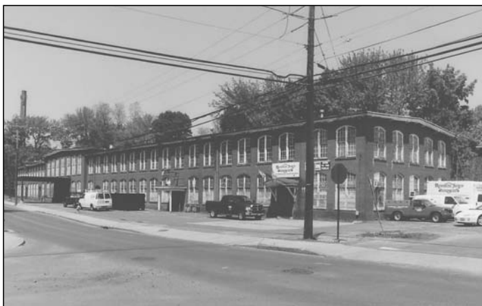
A lot of windows: Some of the 44 windows on the History Center that will be restored (above); one of the windows slated for restoration (right).
