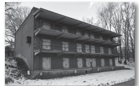
Three level vault building on Elm St. Extension
