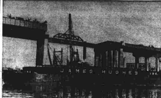
Steel Span Closes Pike Gap 30-ton girder connecting the east and west portions of the Connecticut turnpike bridge over Bridgeport harbor, was set in place today as the Terry Contracting Company, of New York, began closing the last gap in the bridge structure. The harbor bridge is considered the critical point in the
