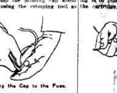
Crimping the Cap to the Fuse. shown in the illustration. Next punch a diagonal bole in the cartridge with the end of the crimping tool, making the cap. Insert the cap into this hole
