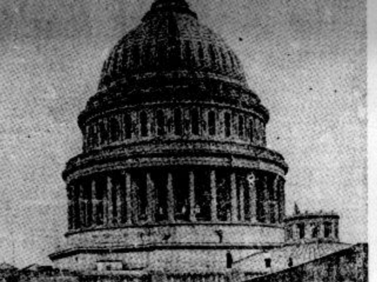
VIEW OF U. S. CAPITOL DURING PAINTING. The dome of the United States Capitol at Washington is kept in excellent condition by painting it every few years.
