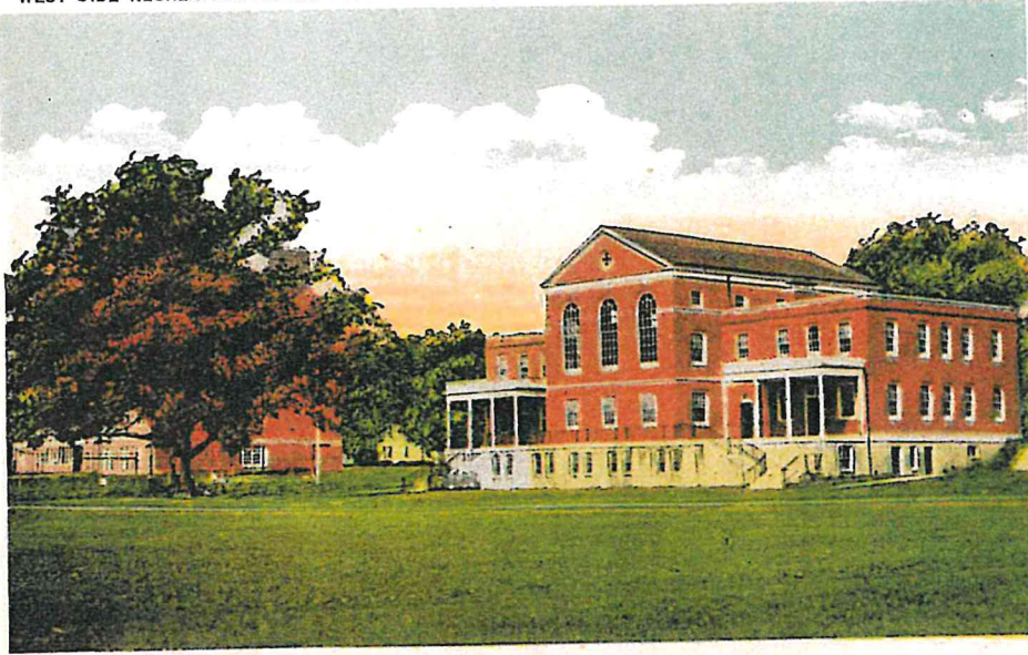
WEST SIDE RECREATION BLDG., SO. MANCHESTER, CONN.
