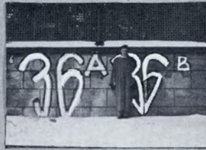
THE OLD WALL
