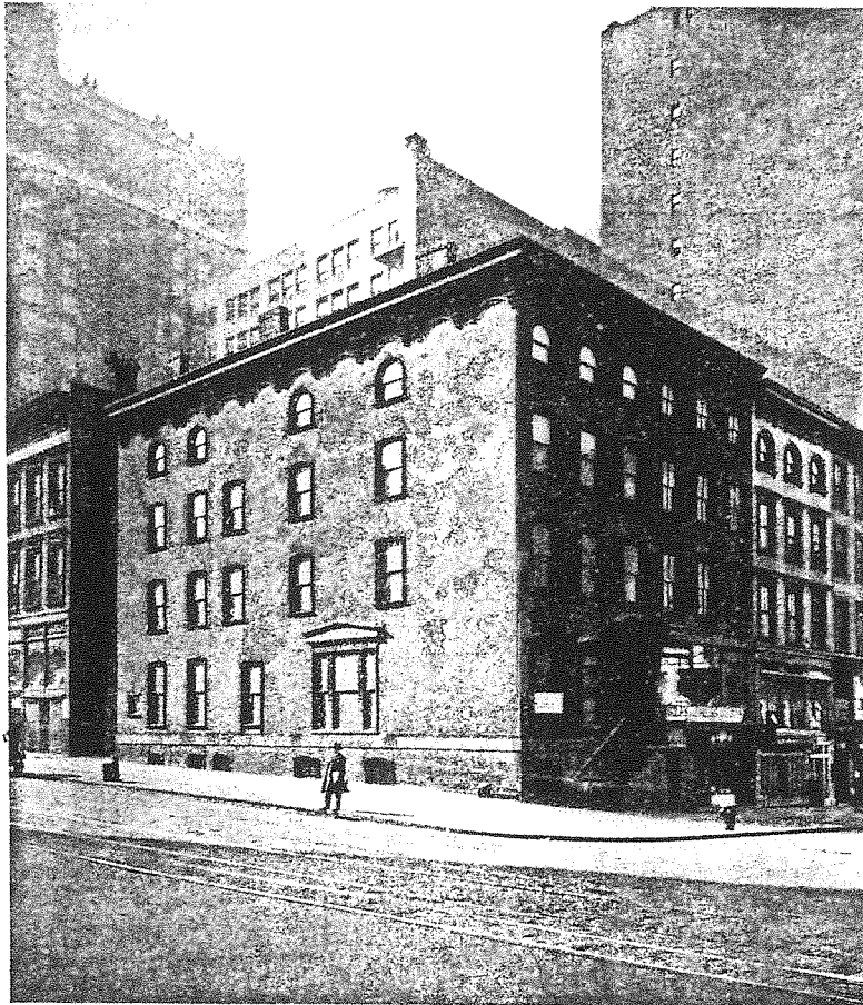
Present corner at Madison Avenue and Thirty-fourth Street on which is to be erected a new building in which Cheney Brothers will have their New York sales rooms when completed next year. This photograph was taken on May 20th.
