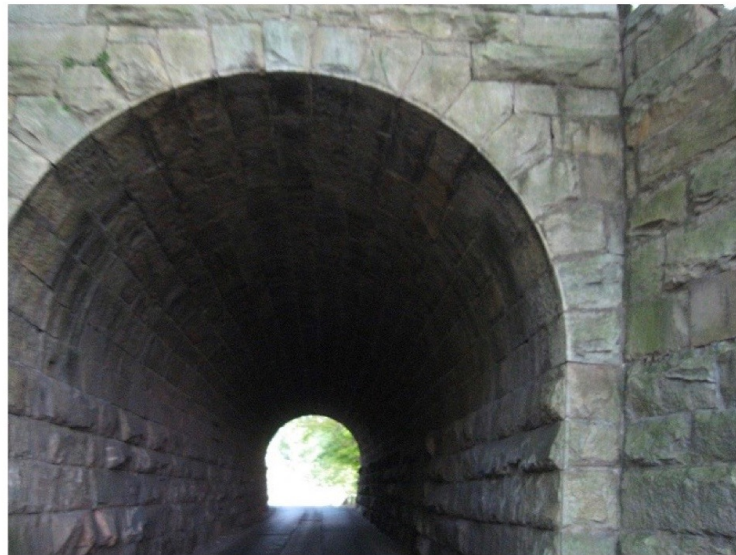
The Vernon Tunnel, which Jeremiah Grady helped to build
