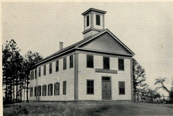
CENTER ACADEMY HOME OF MANCHESTER LODGE 1855 TO 1875 1886 TO 1913
