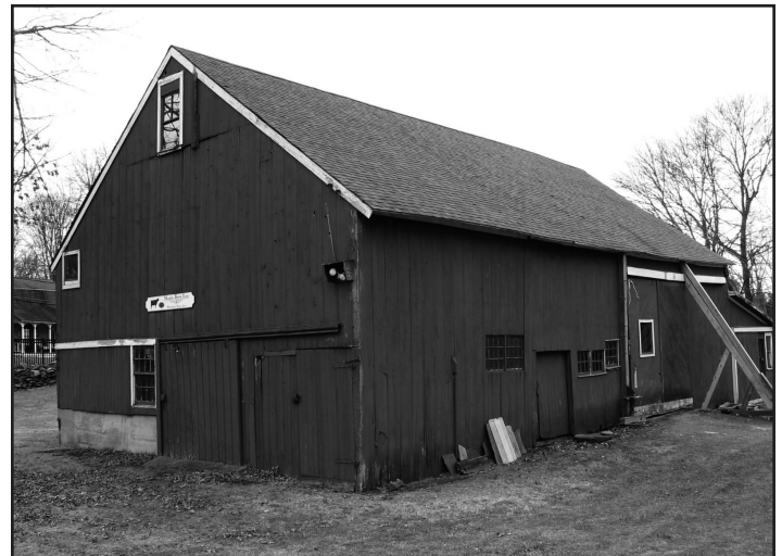
Notice the straight eave line after being repaired
