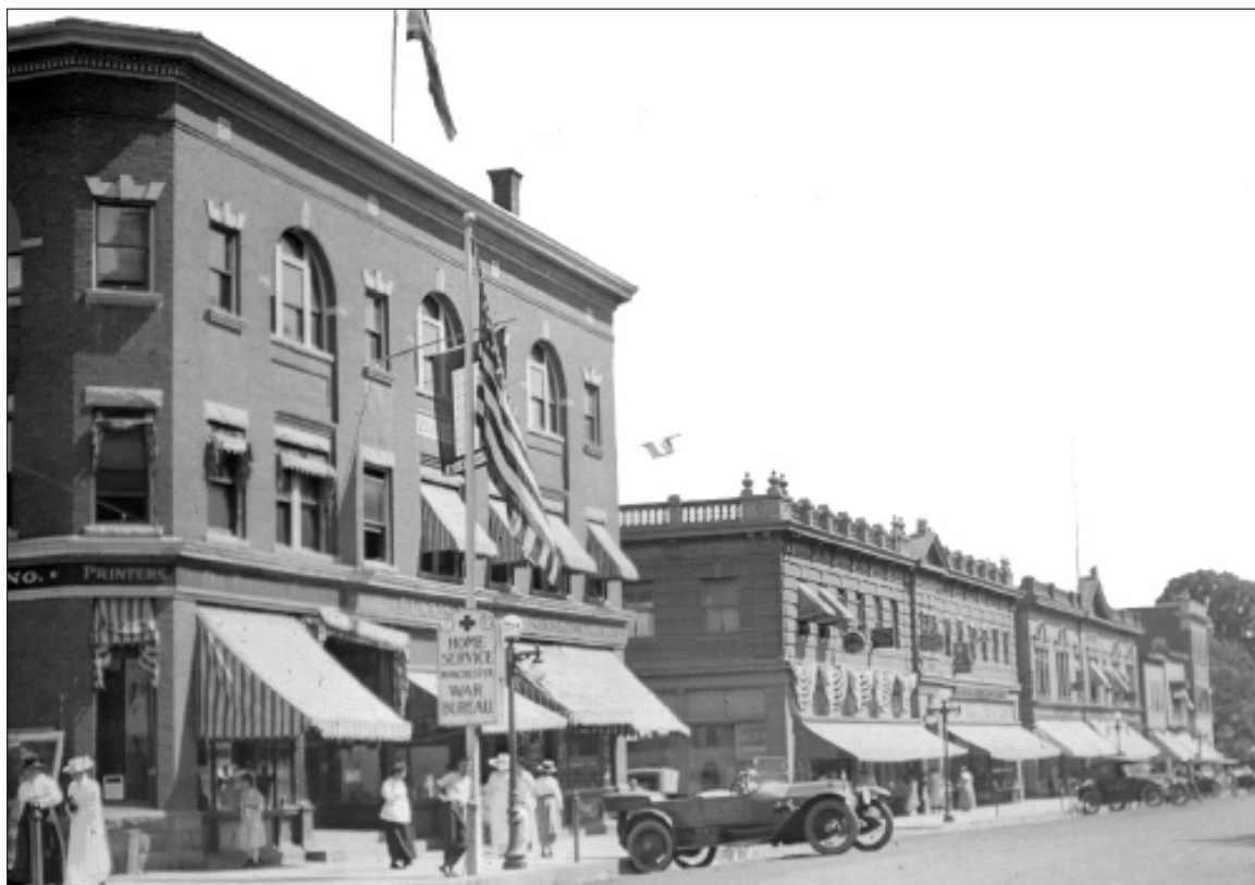
Three-story Ferris Brothers brick building sits on its original location, the corner of Oak and Main Streets. It would be moved east to the corner of Purnell Place and Oak Streets and turned 90 degrees to face Oak when purchased by the Watkins Brothers where it would be joined to their new store. John Knoll photo
