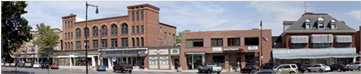
Not much has changed since 1900 along this stretch of Main Street, the Park building, far left, followed by Orford Hall/Hotel, the Orford Annex is replaced by the two-story Bank of America followed by the Weldon block.
