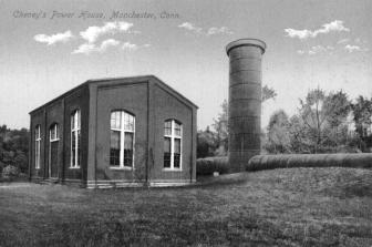
water power harnessed by the dam at Union Pond. They also acquired the site of the former Keeney Paper Mill on North Main St. beside the Hockanum River and converted it to a hydroelectric power station. The electricity generated by the Westinghouse dynamos was transmitted to a substation in the southern part of town and used to power the new velvet mills and carpenter shop.
